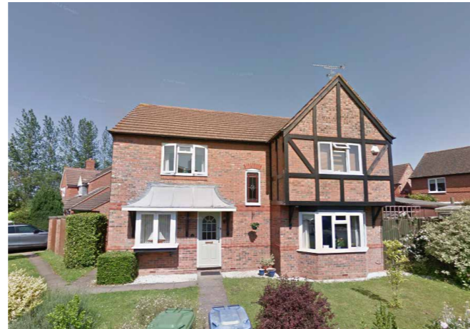
[01] WHITEHEAD DRIVE Detached housing incorporating gables and garages to the side.
