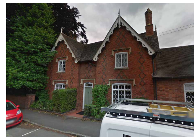
[08] CHAPEL STREET Decorative dark brick detailing to the facade of the building
