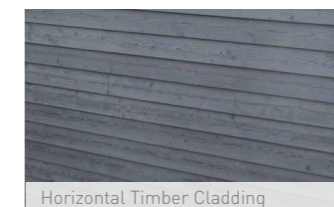
Horizontal Timber Cladding
