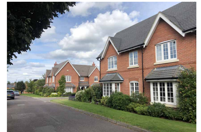
[03] GRANTHAM ROAD A development showing the use of gables and projecting brick courses.
