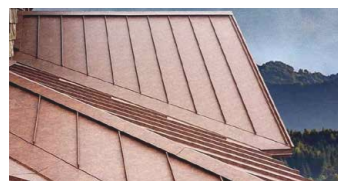
Coloured Steel Roof
