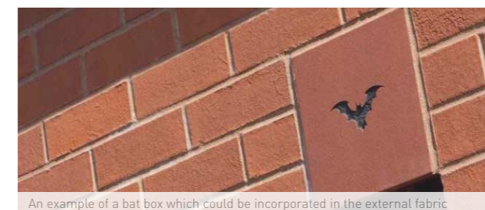
An example of a bat box which could be incorporated in the external fabric
