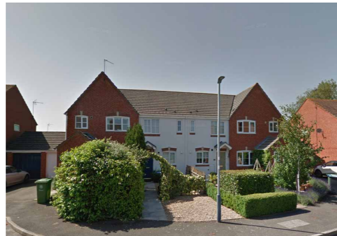
[04] WHITEHEAD DRIVE Semi-detached housing incorporating two material finishes to the facade.
